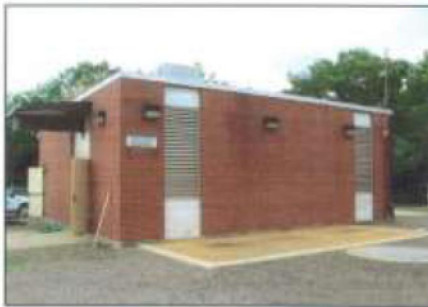
Prairie Creek Lift Station
